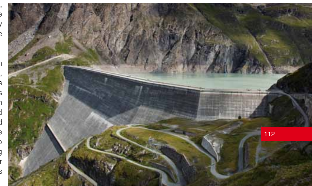
Grande Dixence Dam, the tallest gravity dam in the world, supplies hydroelectric power for 400'000 Swiss households
