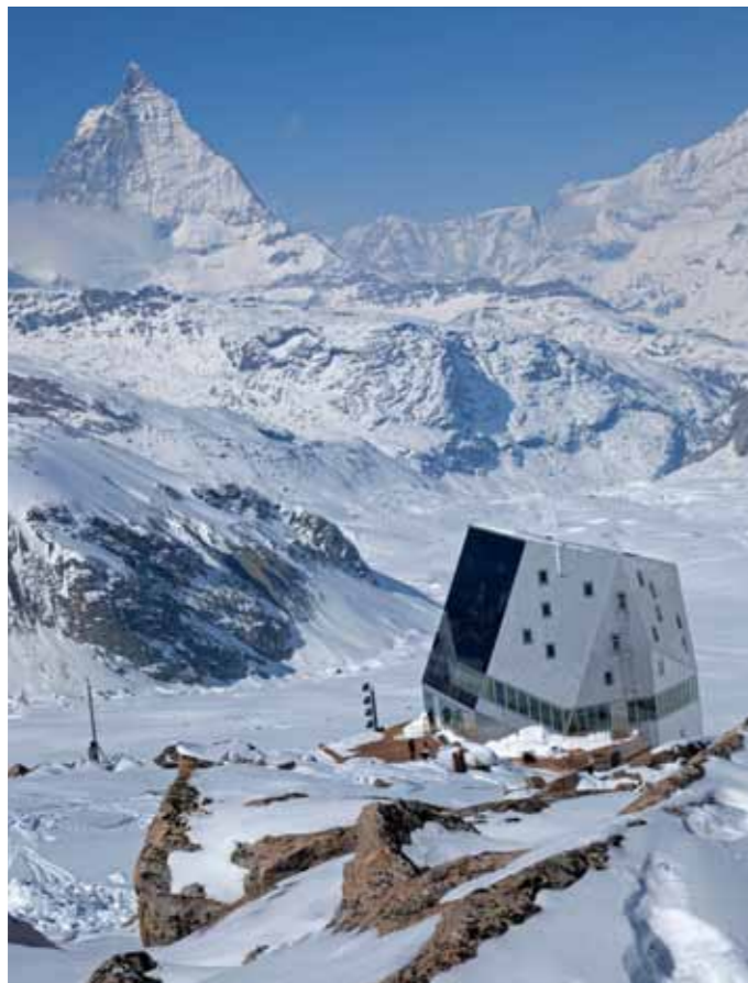
The Monte-Rosa-hut, located in the Swiss Alps at 2883 meters, was built in 2009. It is designed to obtain 90 % of its power needs from the sun thanks to its ultra-modern photovoltaic system. The water is produced from melting glaciers then collected and stored in a large reservoir 40 meters above the hut. Bands of windows allow the sun to heat air inside the spiral building with the redistribution of thermal energy produced by visitors. Over the next few years, the hut will become a research station for the students from the ETH Zurich. They will use it to investigate how to use energy and resources efficiently. An exhibition on the new Monte-Rosa-hut was shown at Yonsei University in April 2011.
