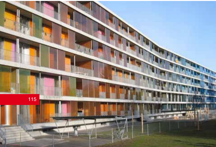
A colorful example of a Swiss made low-energy-consumption building: a MINERGIE-ECO® house in Zurich. Underneath the bright and cheerful façade, it hides a secret: a 20-cm thick isolation layer that saves considerable energy by keeping the heat firmly locked in. It is also connected to an environmentally-friendly district heating network that recovers the heat generated by a local household waste incinerator.
